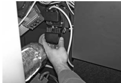
Fig. 154 Disconnecting the blower plug
