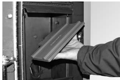
Fig. 128 Removing and cleaning the baffle plate
