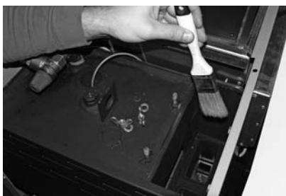
Fig. 146 Cleaning top heating surfaces and linkage
