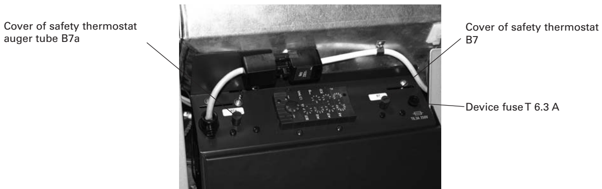
Fig. 163 FireWIN control panel, rear right side panel removed
