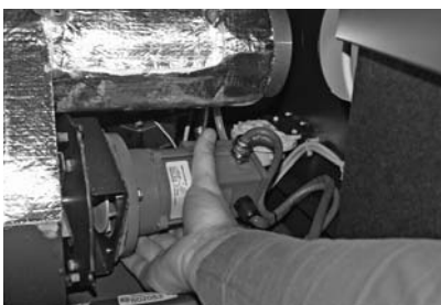
Fig. 155 Removing wing nuts, removing the blower unit
