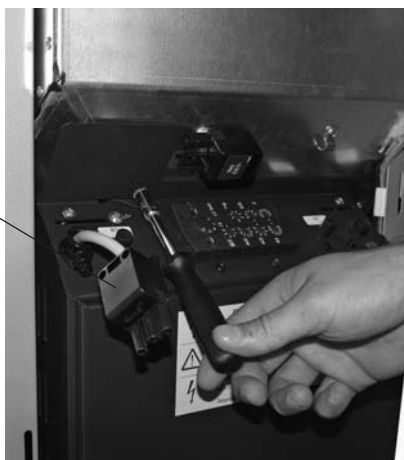
Fig. 30 Disconnecting the mains power plug and removing the screw.
