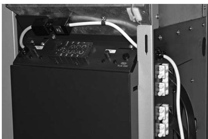
Fig. 29 Cable feed-throughs – rear view
