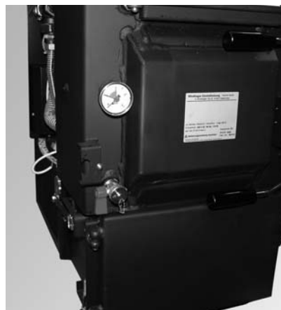
Fig. 16 Screwing pressure gauge into shut-off valve
